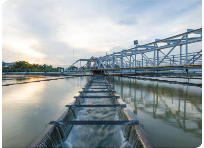
Prevent the growth of biofouling on the weirs and walls of the clarifier
